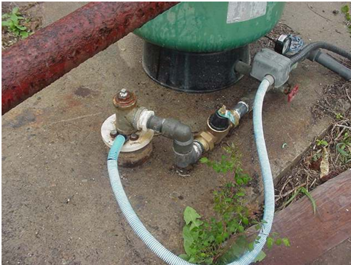
Picture of typical installation PUMP STOP VALVE
